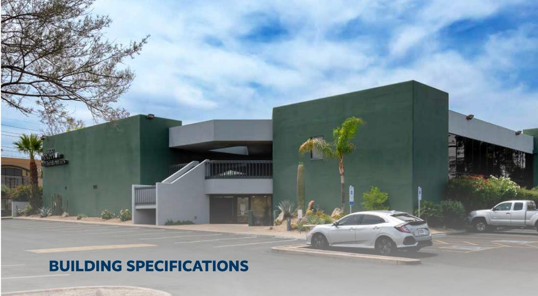
**GENERAL CONSTRUCTION:** Two-story with structural steel columns, CMU masonry block and parapet style roof.
